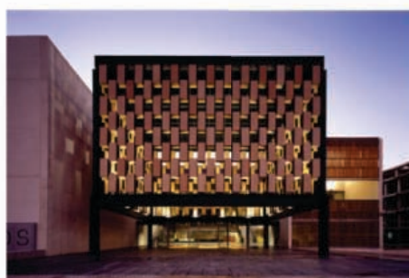
Figure 13: Fireproof ceramic element glued to steel column and clay façade elements in the Convention centre of Peñíscola
